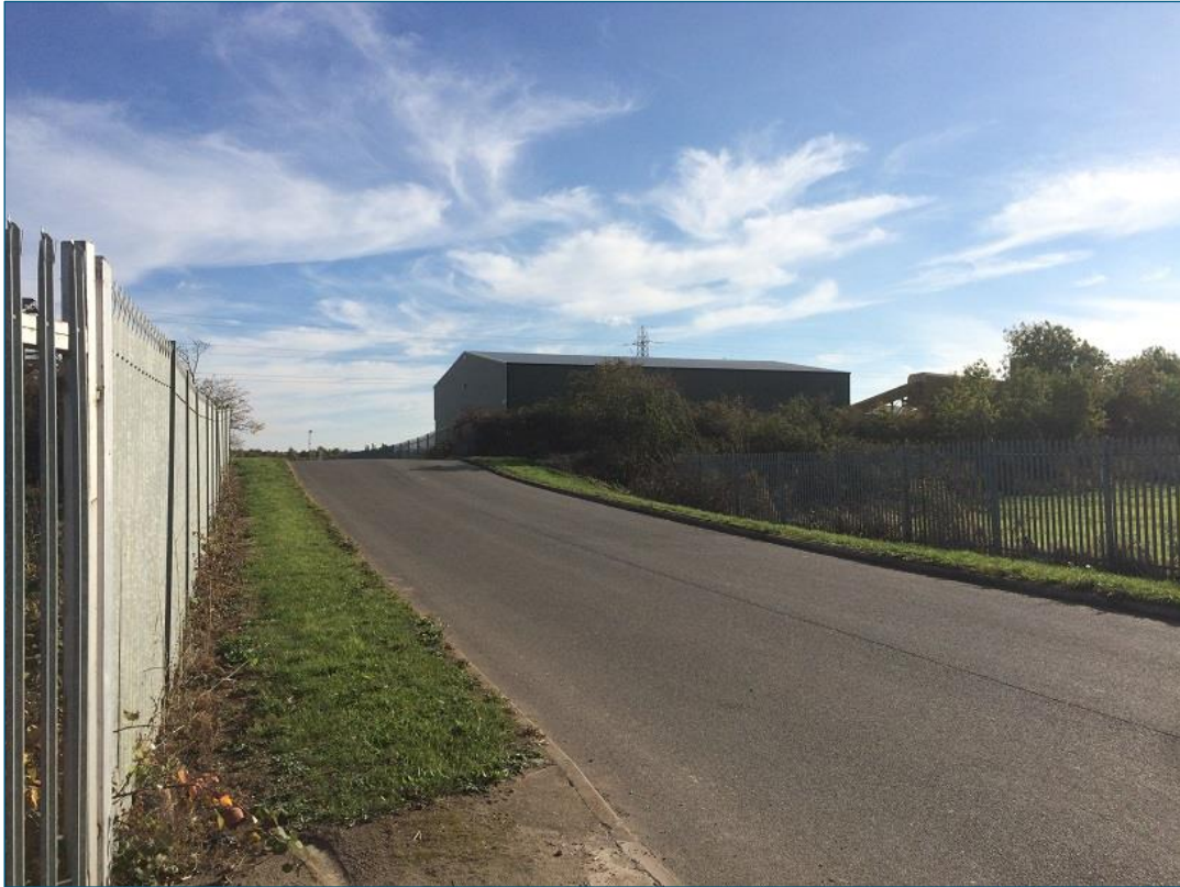
Plate A8.1.6 View of the Roman Bank and New Road Traversing over it, Looking East
