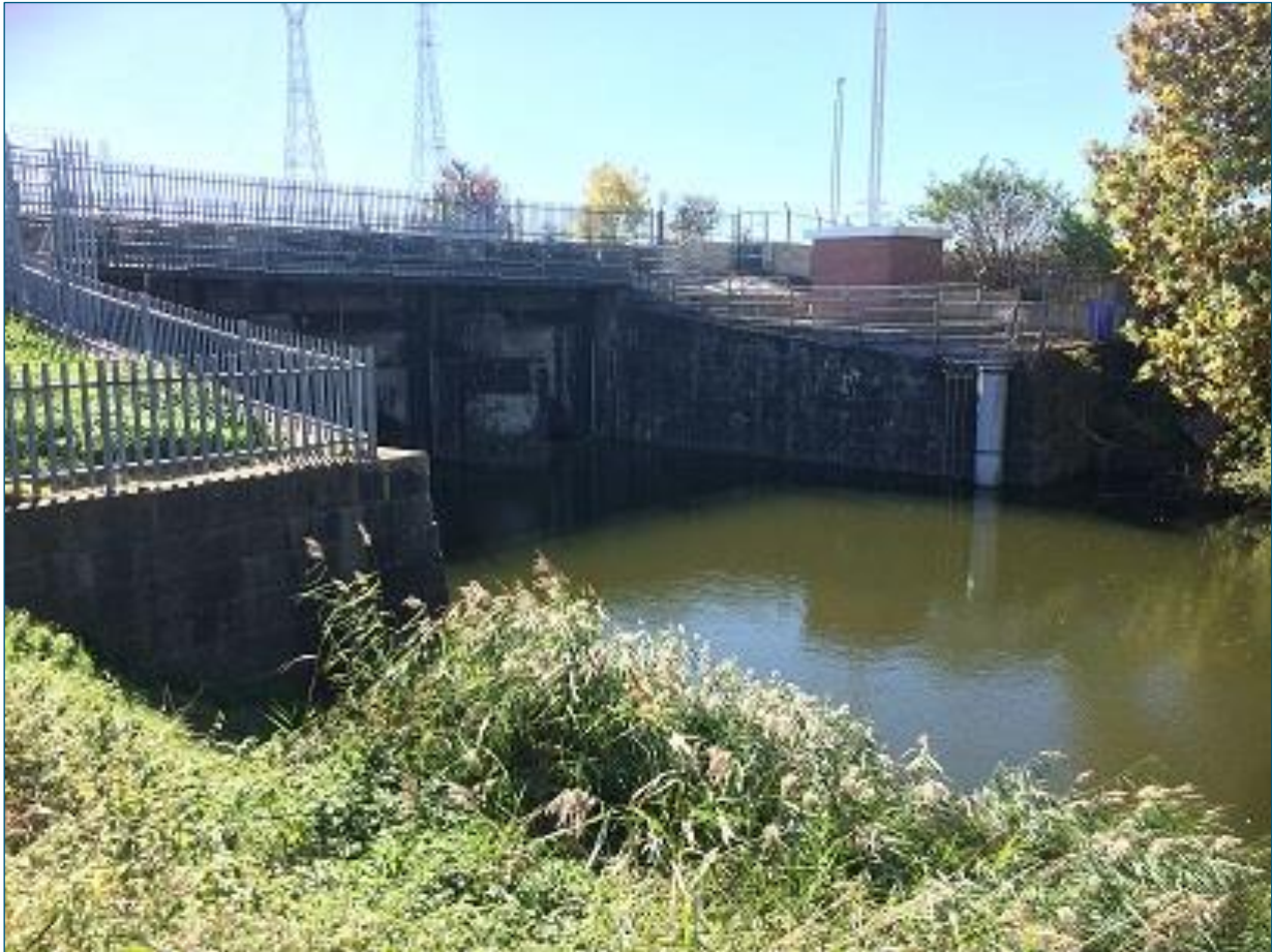
Plate A8.1.16 Maud Foster Sluice, view from Windsor Bank, Looking South-west
