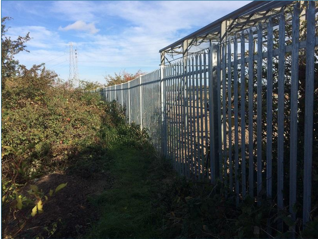
Plate A8.1.7 View Down the Roman Bank Footpath, Looking North-west. Note Fencing on top of Bank
